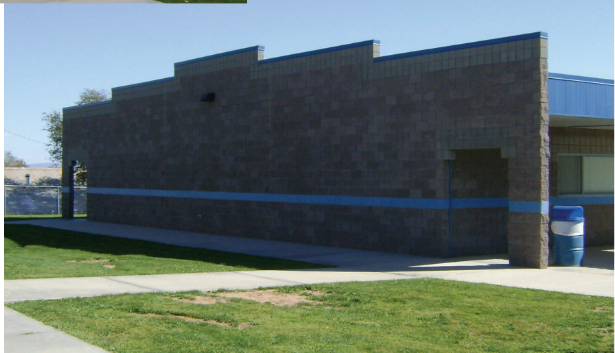
Sealed split-faced block—After
