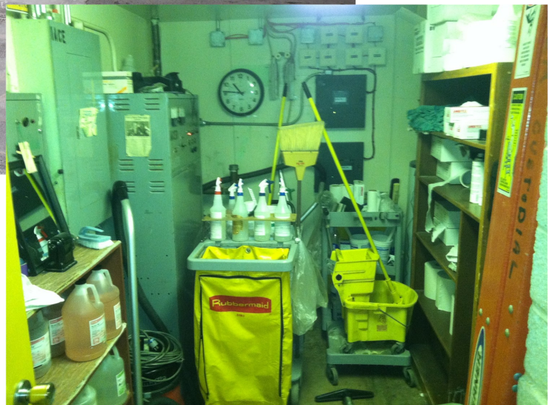
Inappropriate storage in mechanical rooms.
